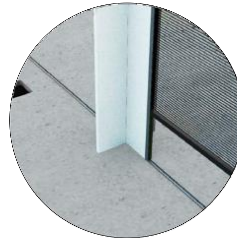
COLUMNS WITH INTEGRATED PROFILES FOR ROLLERS
