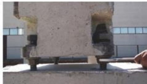
All the concrete elements are joined by bolted steel connections, all reversible reusable in the future.
