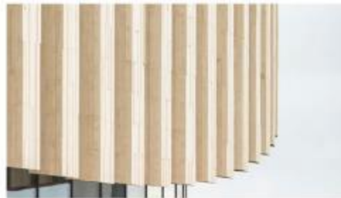
Bio-treated timber used in large scale on an arena in Copenhagen, Denmark.
