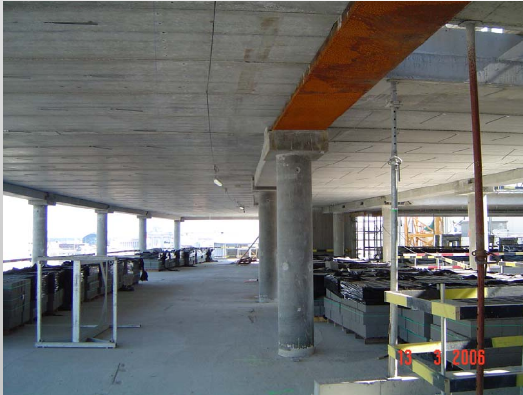
HC on bottom fange steel beam
