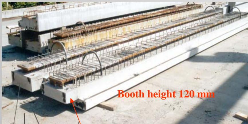
Beam end with half joint
