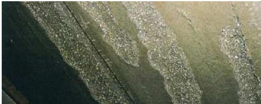
*Due to concrete exposure to fire, free water in the concrete changes phase to steam. If the steam is not released through concrete due to its dense packing then it causes pieces breaking off: explosive spalling.*
