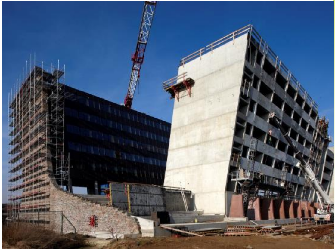
Office building with thermal activated floors – Hasselt - Belgium
