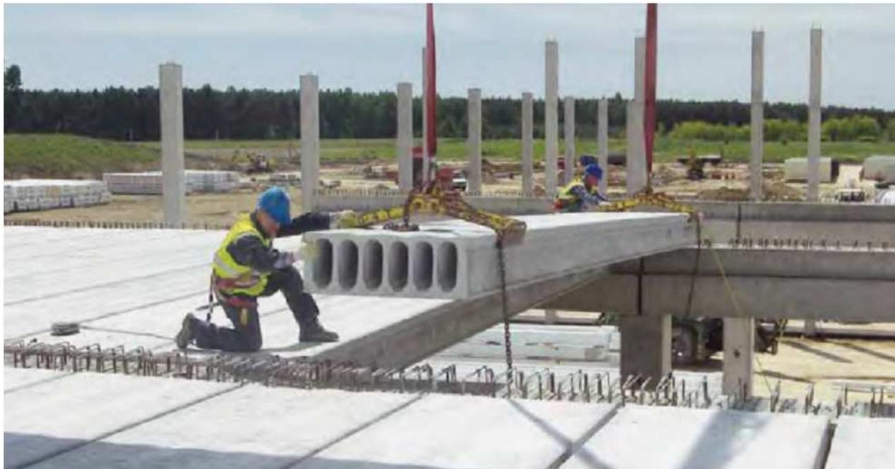
HC floor slabs can also be constructed with restrained support conditions, especially in combination with cast in-situ beams and walls, or in composite structures.
