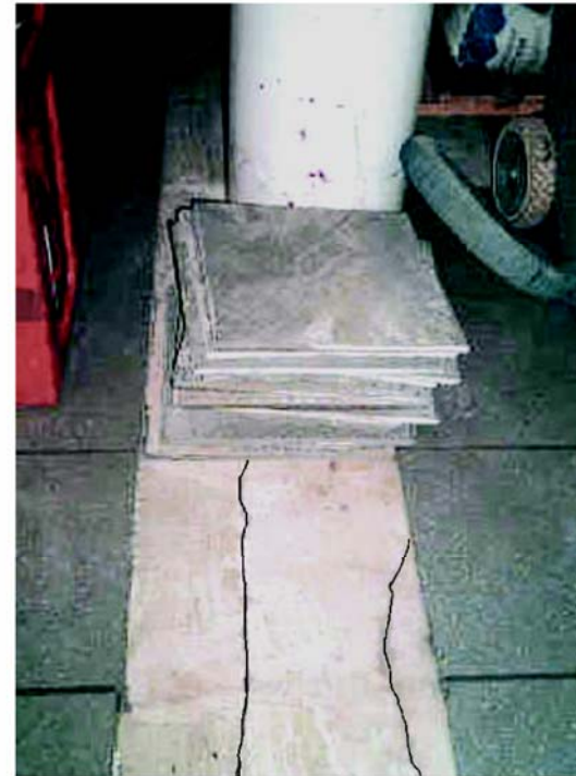
Typical cracking HSQ (hat beam)
