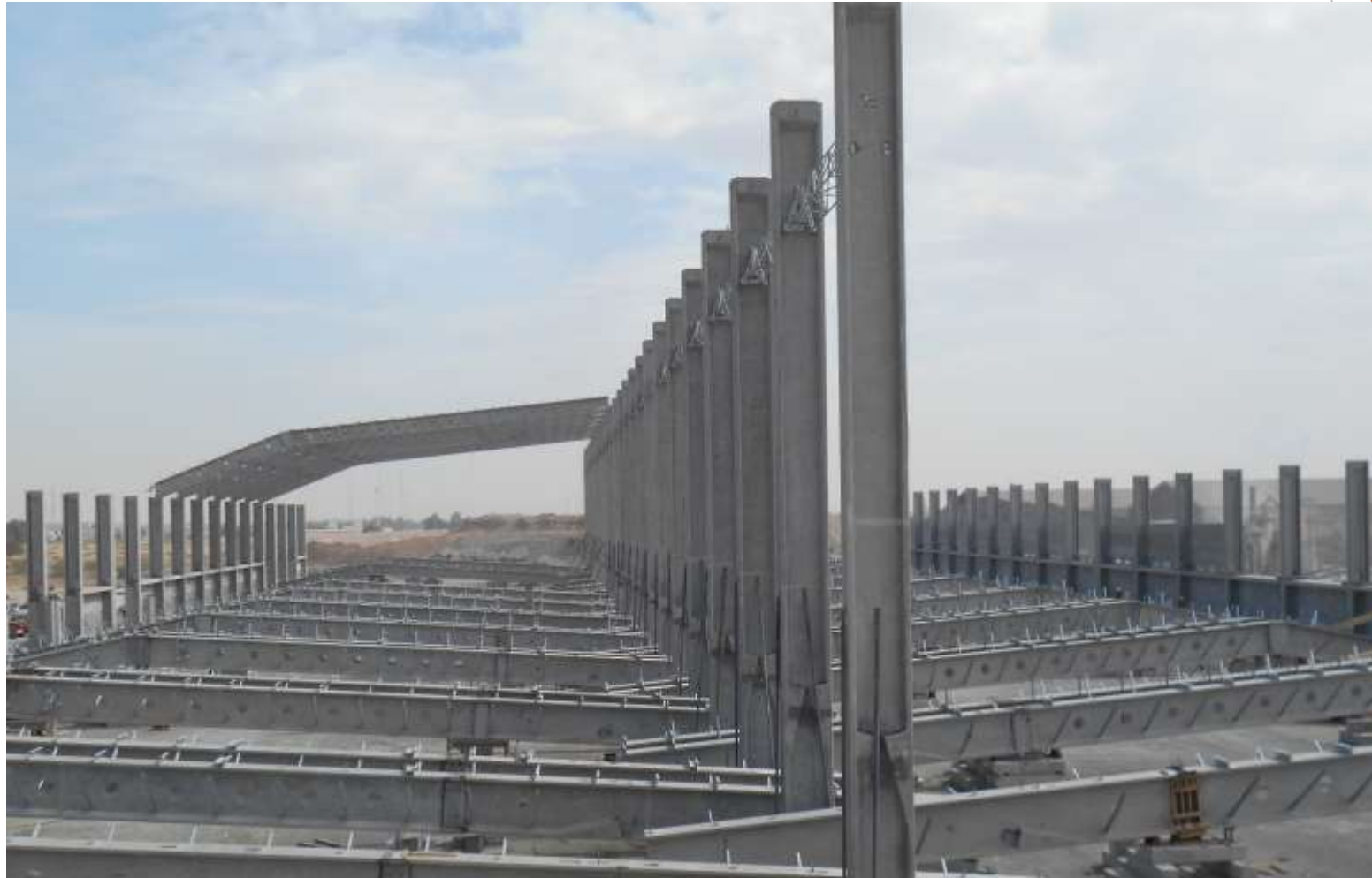
Sharjah Cement Clinker Shed- Hollowcore Retaining Walls
