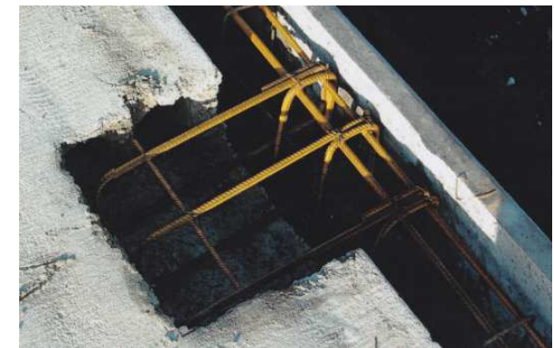
Shear connectors A_{s5}
