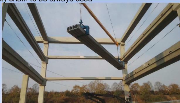
Photos of H.C. slabs erection (H 420 and L>15 mt). Three-story building (100.000 m2 tot ) for Amazon logistic center
