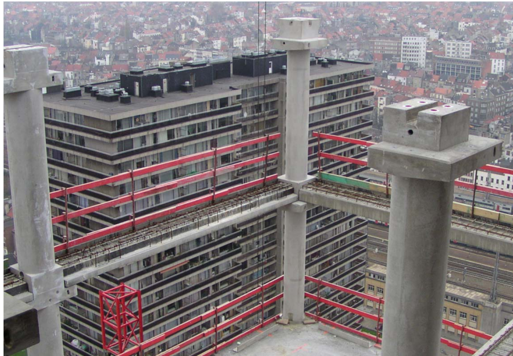
Sleeves in columns for passage of ties
