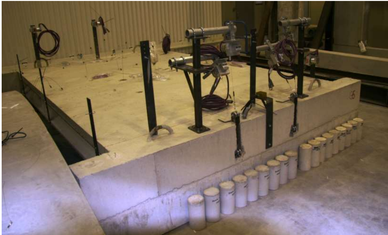
Finished test floor G5 with complete measuring equipment
