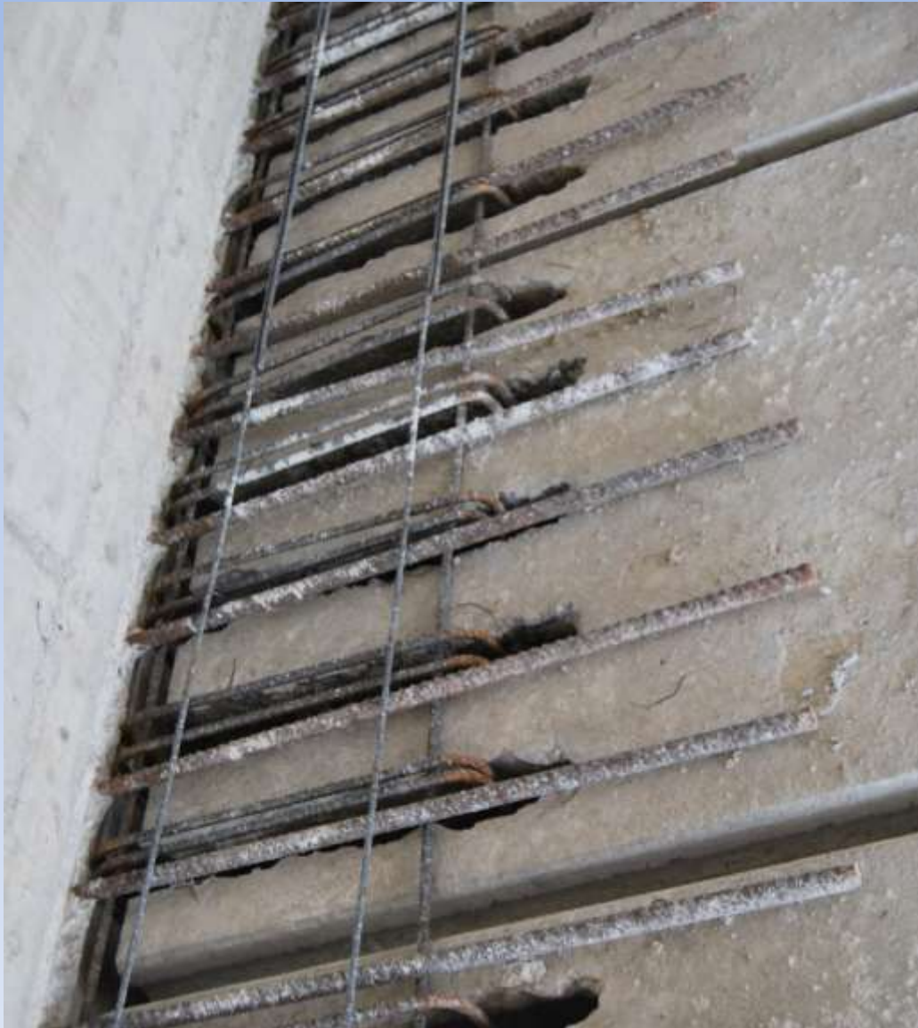
Detail of collectors between hollow core slabs and shear wall
