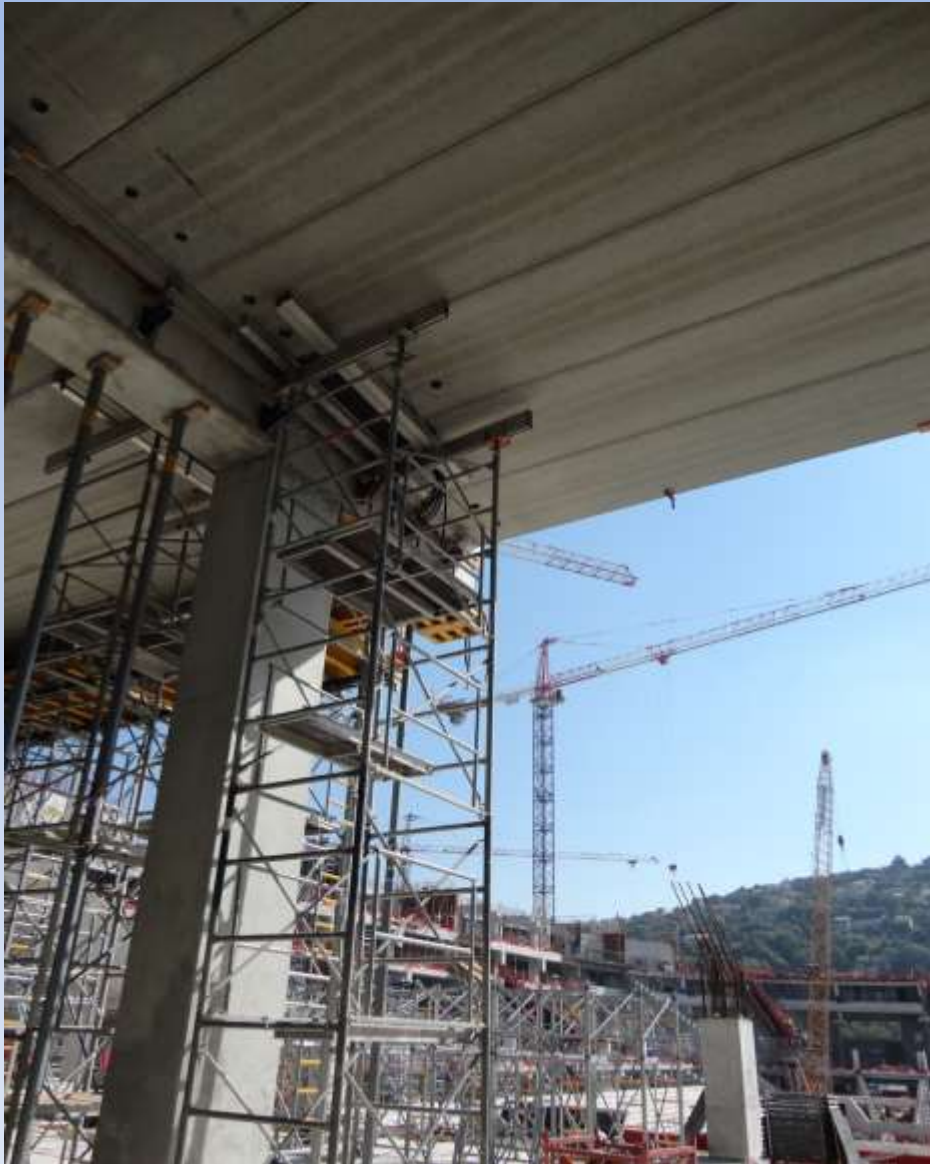
Hollow core slabs for the erection of the Nice Allianz Arena, Nice - France
