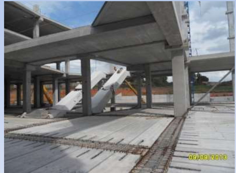
Detail of use of hollow core slabs for irregular shape floors, Rome - Italy
